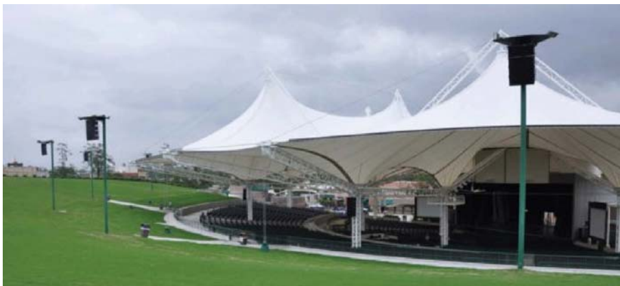
The lawn at the Cynthia Woods Mitchell Pavilion is addressed by an EV XLC system comprising 32 XLCi127DVX and eight XLCi907DVX line array loudspeakers, mounted in various configurations on a total of nine posts.
