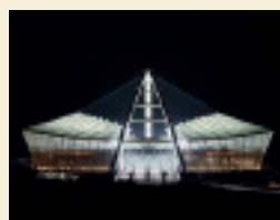
Moses Mabhida Stadium (Architects: von Gerkan, Marg and Partners. Photo: Marcus Bredt)
