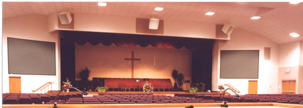
3 White Electro-Voice FRX-940 loudspeakers cover the sanctuary at Montandon
