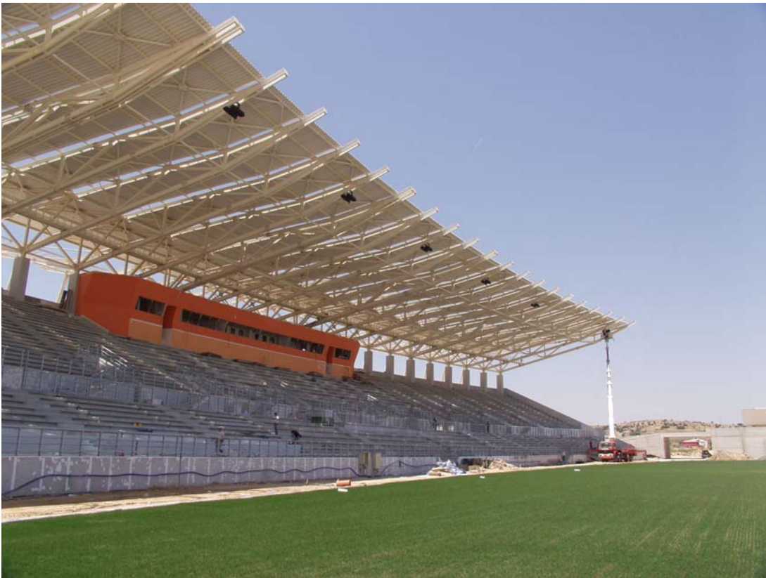
The new sound system for the Equestrian Olympic Center in Markopoulo, near Athens. The first sound system installed for the 2004 Olympic Games.
