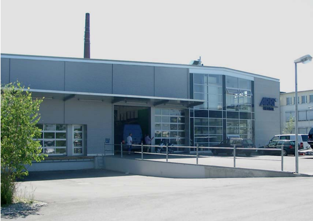
The new ARRI Rental headquarters in Ismaning, near Munich
