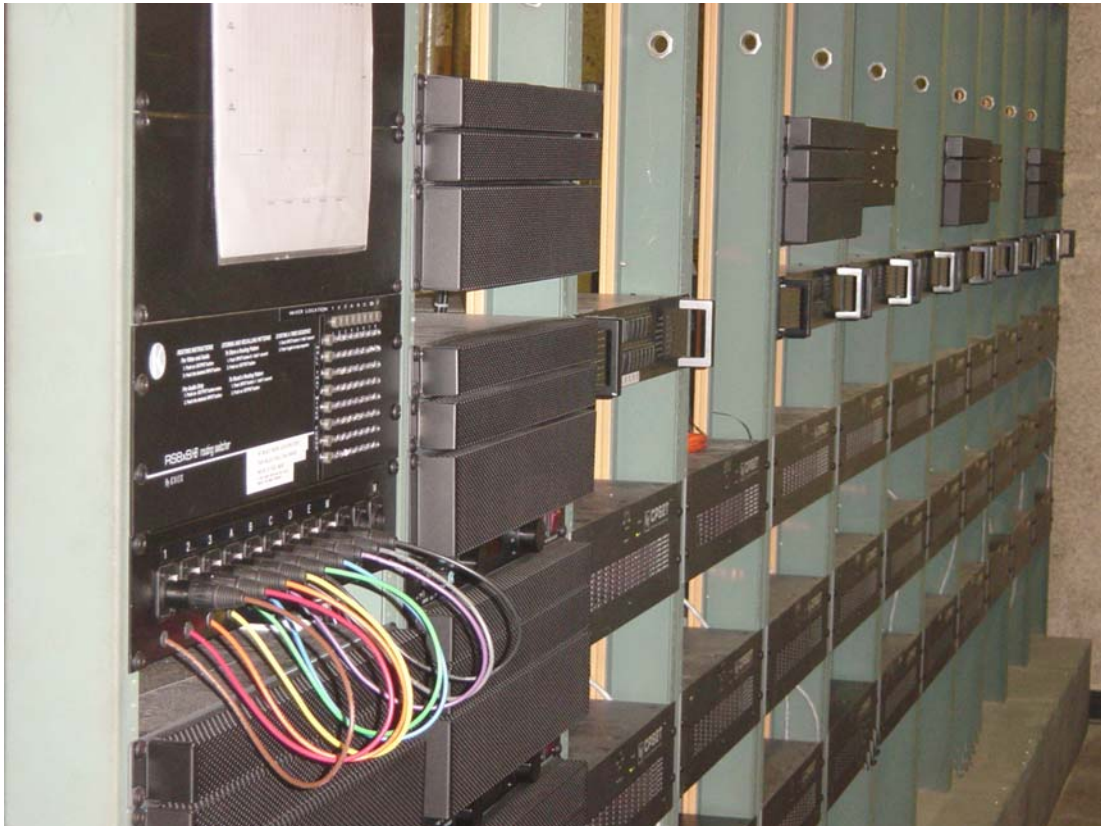
A color-coded routing switcher keeps patching simple for end-users at the Cox Convention Center
